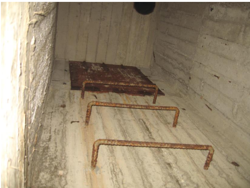
Vertical shaft (5 m climb) and the cover whose bolts need to be detached.
