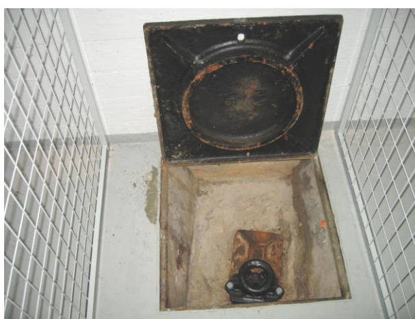
Repaired and serviced sewer shutoff valve.
