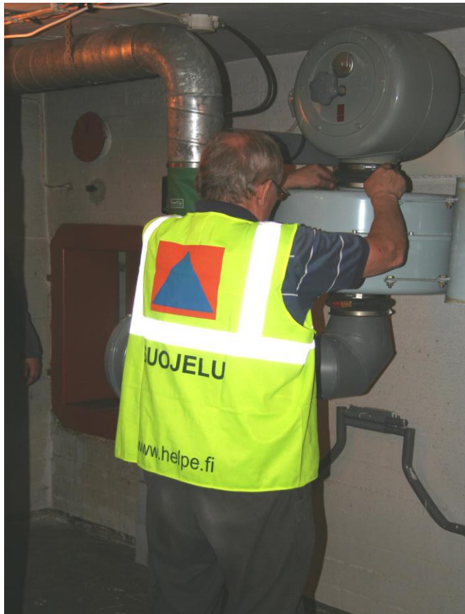
Installing the filter.
