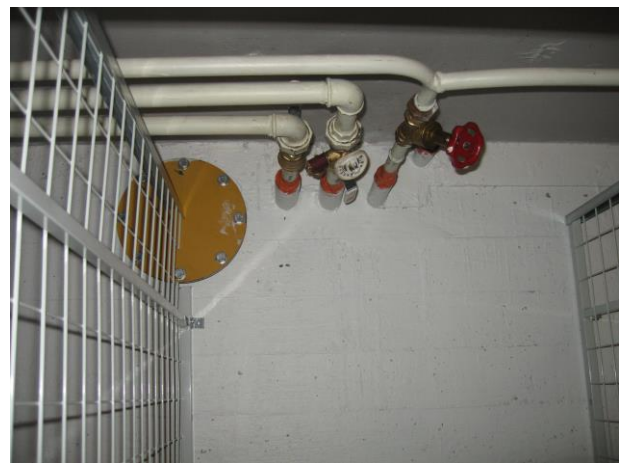
Sealing the lead-throughs with tape.
