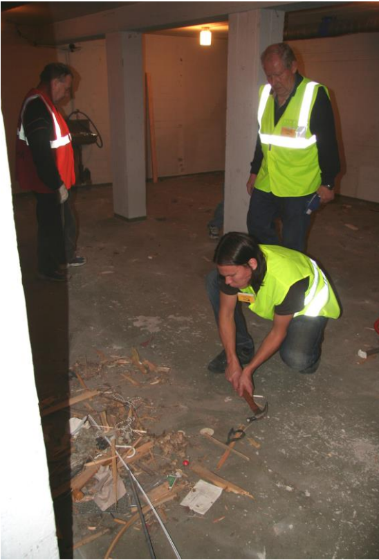
Removing steel nails from the floor.
